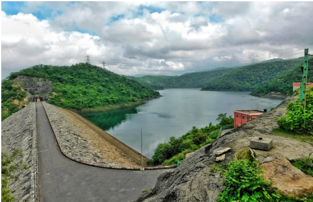
Photo 51. Lower dam of Purulia.
