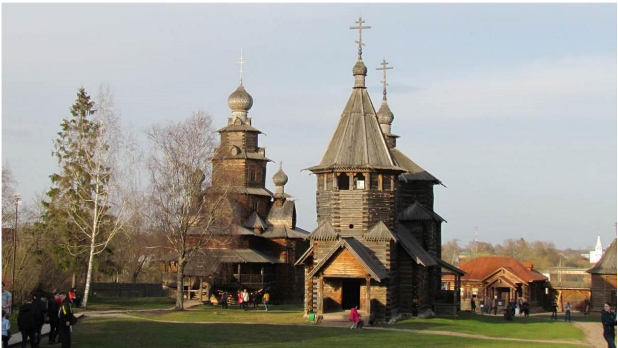
Photo 36. Its most famous exhibit is the Church of Saint Nicholas, dating from 1766, which features a log structure and a distinctive shatyor (octagonal pyramid) roof. Suzdal, Russia.
