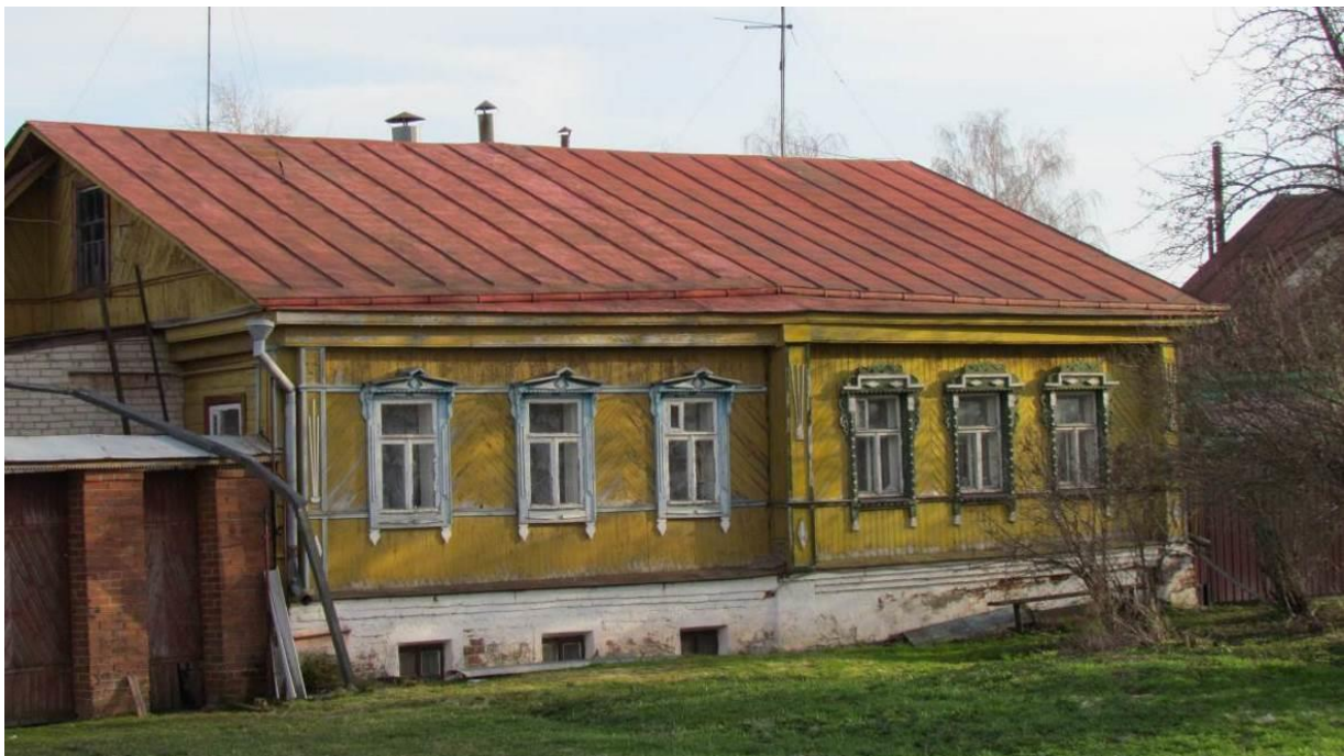
Photo 28. Izbas are traditional wooden houses decorated with carved window frames and colorful folk motifs. Suzdal, Russia.
