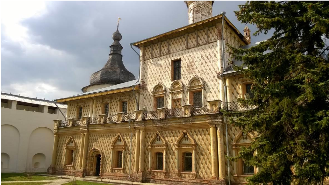
Photo 81. Church of Hodegetria is a building in the style of the Moscow baroque. The facade is decorated in the technique of diamond rust: diamond-shaped volumetric cladding. Rostov Kremlin, Russia.
